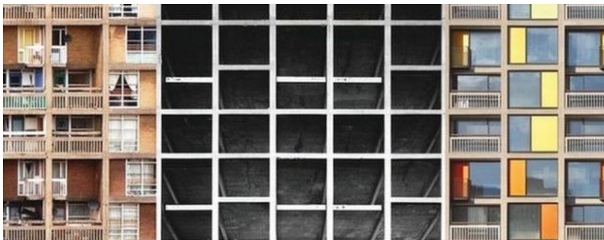
Figure 5 – From the left section of the non-renovated complex; section from the structural cage; section from the redeveloped building with the inversion of opaque / transparent proportions © Hawkins / Brown.
